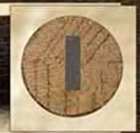
Inner Pole Reinforcement
